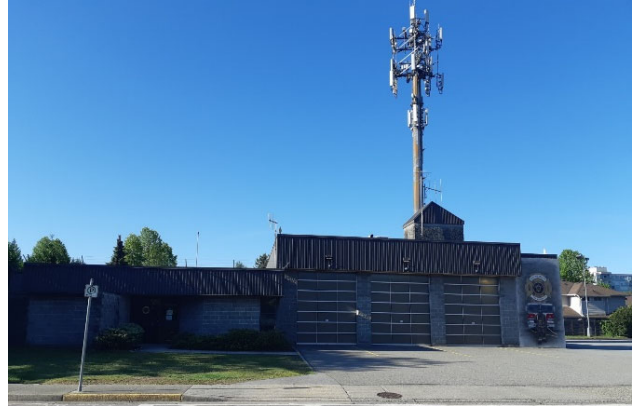
Figure 1: Existing Fire Hall
