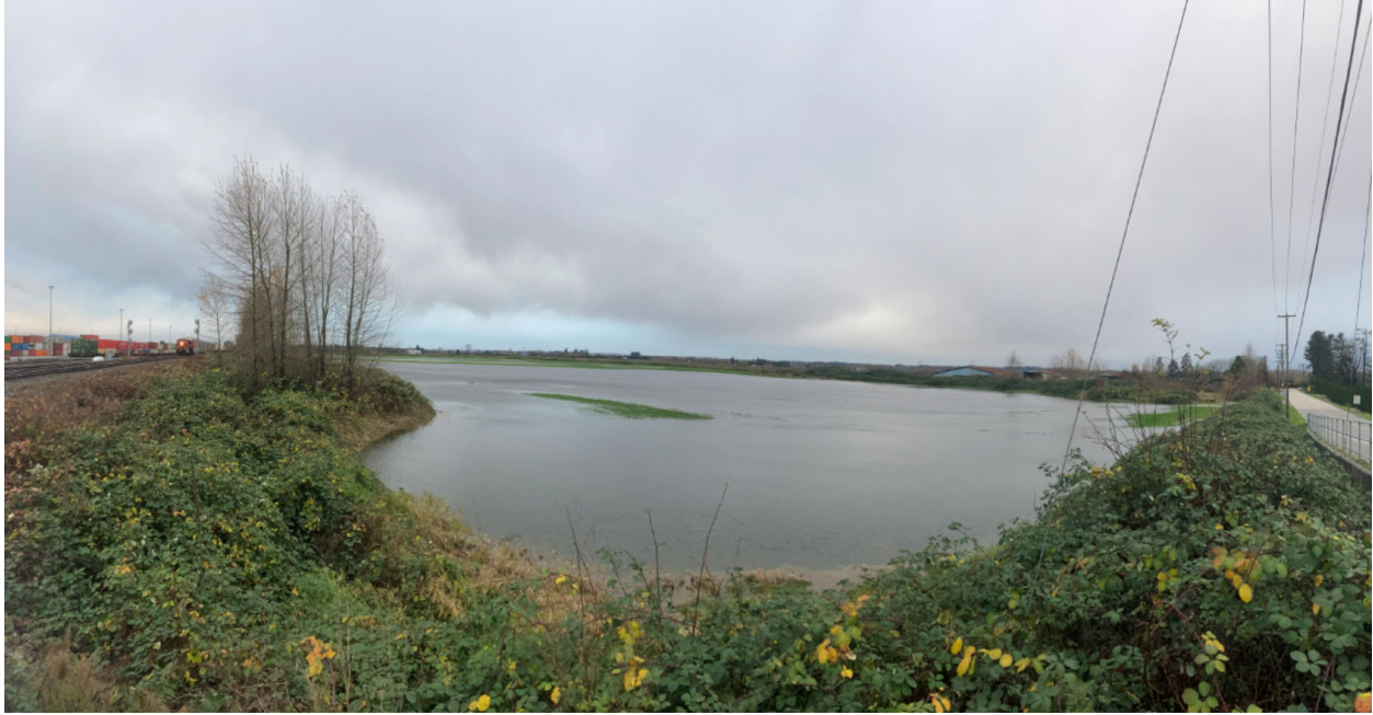
Figure 5 – Flooding at Proposed Project Site, November 15, 2021
