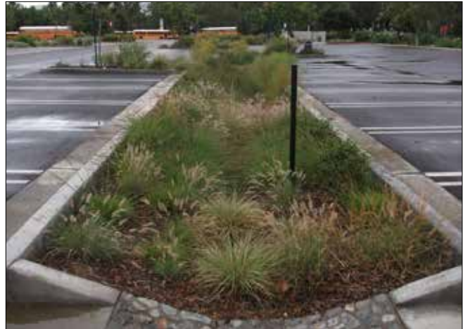
Planted island allowing surface water infiltration
