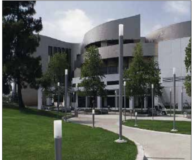
Unified family of lighting fixtures
