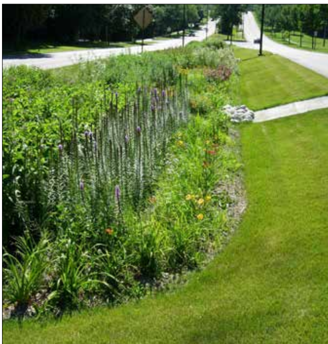
Naturalized swale enhancing infiltration
