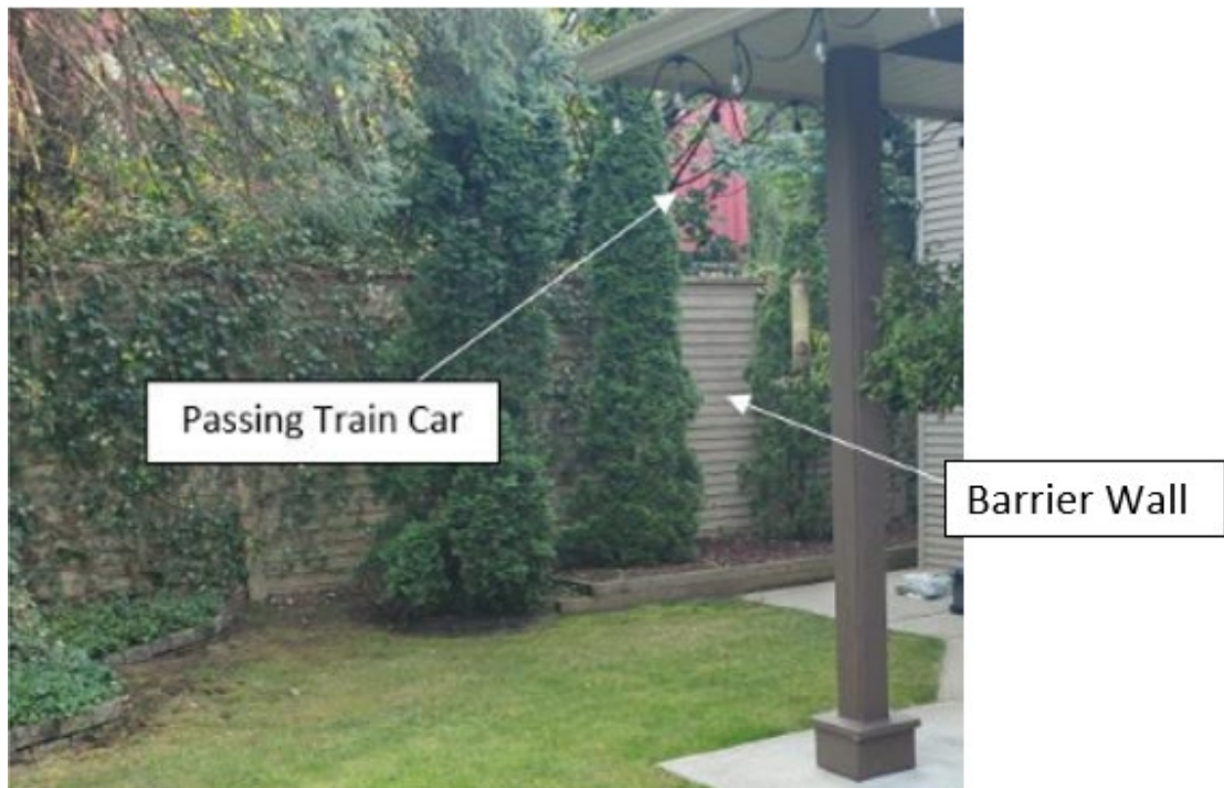
Picture 2: Barrier wall at McMyn Ave. Barriers must break the line-of-sight between source and receiver to be effective.
