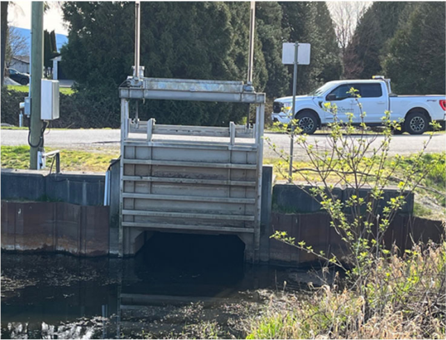
Sluice gate on Hale Rd
