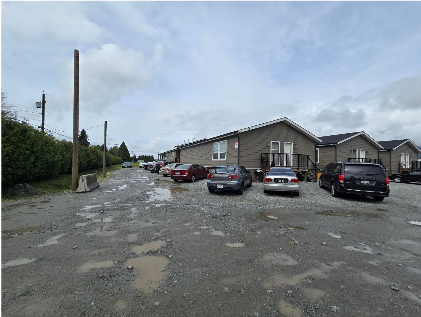
Figure 4: Existing Migrant Worker Housing at Hollandia Greenhouses: View Northwest at Access from Richardson Road
