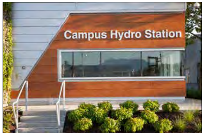
Example – building signage
