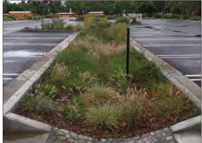
Planted island allowing surface water infiltration
