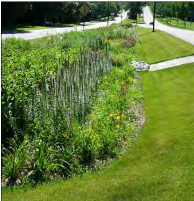
Naturalized swale enhancing infiltration
